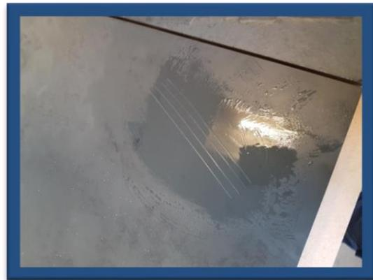
B: Starting with the coarser grit paper (240, although lower grits of around 100 can be used for deeper blemishes or quicker stock removal), sand the scratches and the surrounding area in a circular motion, until the scratch is no longer visible.
