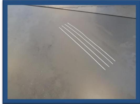
A: Wash the scratches with clean water. You can allow the tile to dry but the following process can be done while the surface is still damp.
