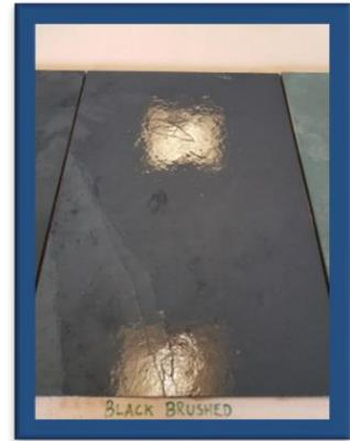
B: After an hour, remove any excess sealer that remains and buff with a microfiber cloth. Tiles should be left for a further 12 hours before applying the grout.
